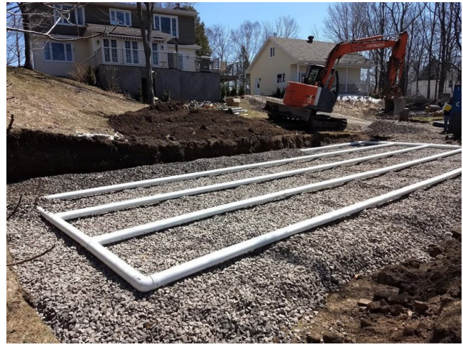
Figure 3: Conventional septic drain field (Source: Nonztp, 2019)
