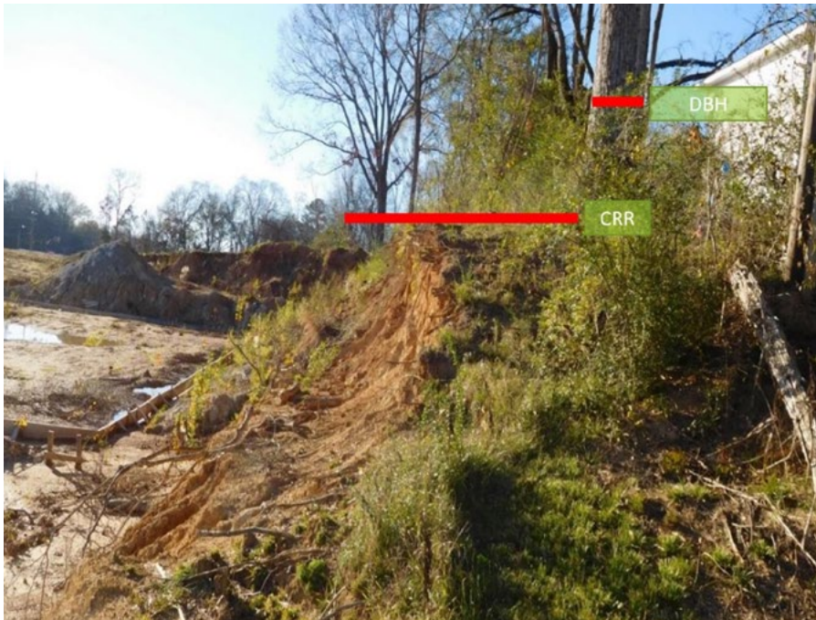
Figure 17: Site disturbance. The construction interfered with the critical root zone as determined by the diameter of the tree (dbh) and the critical root radius (CRR).
